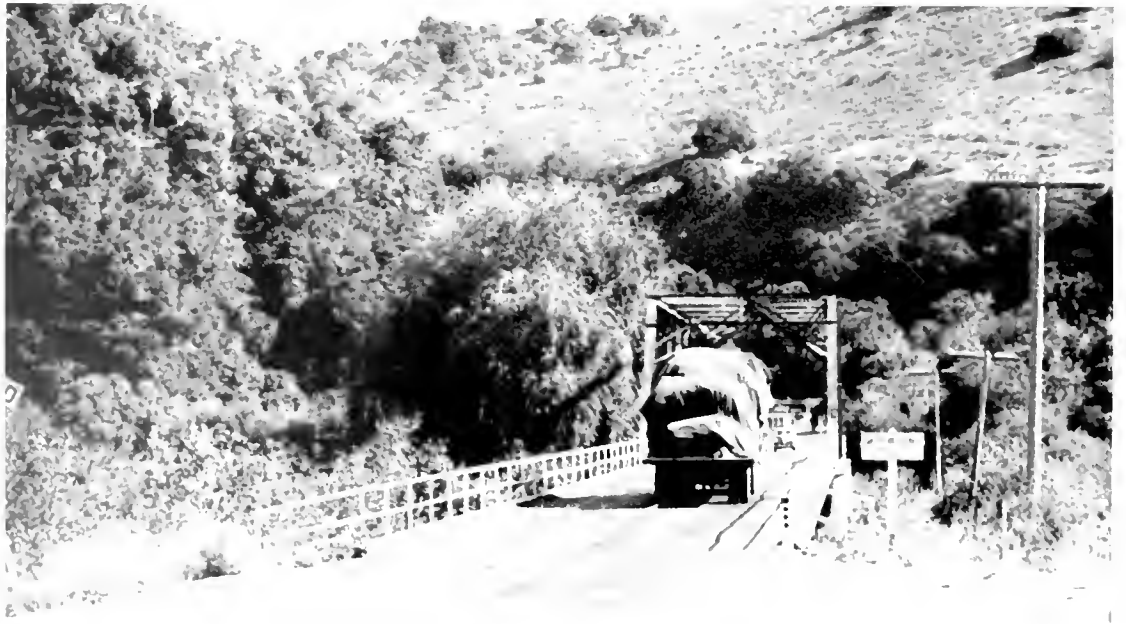
Existing bridge is an old, narrow through-truss steel structure
